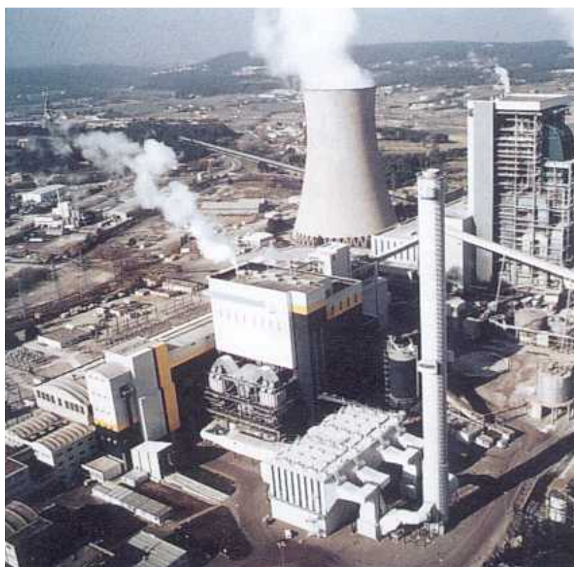
Figure 6: Gardanne CFBC power plant
