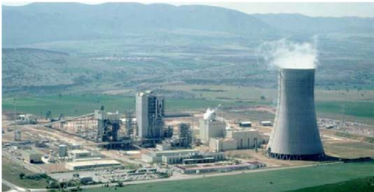
Figure 8: Puertollano IGCC power plant
