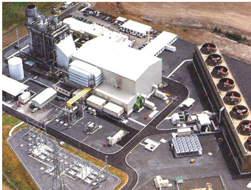
Figure: Combined Cycle Power Plant
