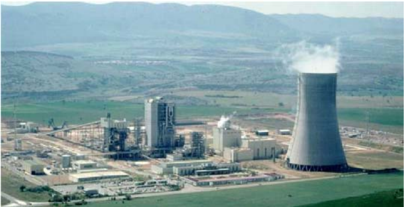
Figure: 330 MWe Puertollano IGCC power plant (courtesy of ELCOGAS)
