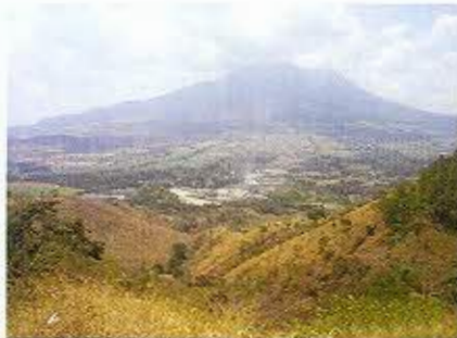
San Vicente Geothermal Field
