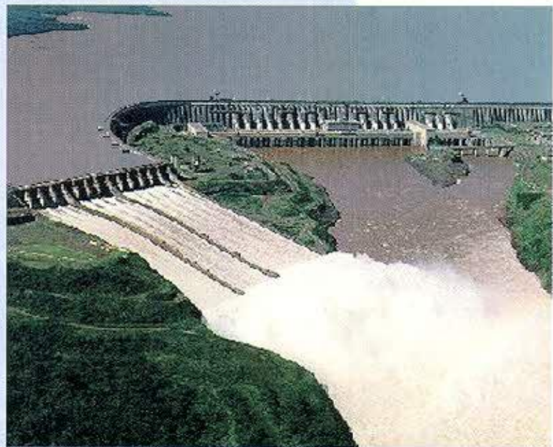
Hydropower station of Itaipú, the world's largest binational project, involving Brazil and Paraguay and whose installed capacity amounts to 12.5 million kW.
