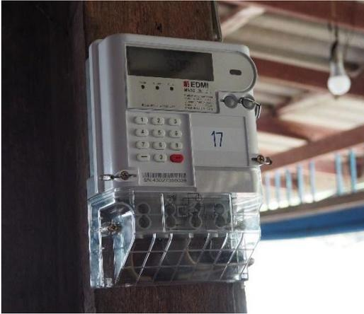
tion (STS) encrypted codes) using keypads on the meter. The meter's LED screen shows the amount of remaining credits (kWh) and has a built-in relay to disconnect power supply once the credits have been used up.
