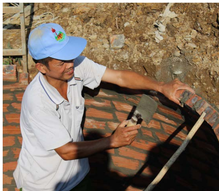
Biogas digester construction in Viet Nam
