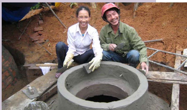
Biogas digester construction in Viet Nam
