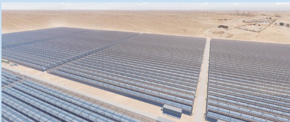
Figure 13: PICTURE OF THE SOLAR-POWERED EOR PROJECT IN OMAN
