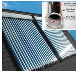
b) Evacuated tube collectors (inset: tube used)
