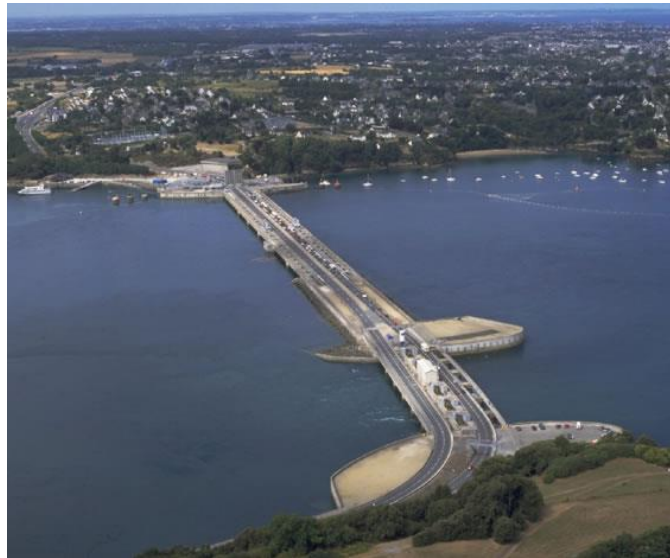
FIGURE 7: LA RANCE TIDAL RANGE BARRAGE IN FRANCE
